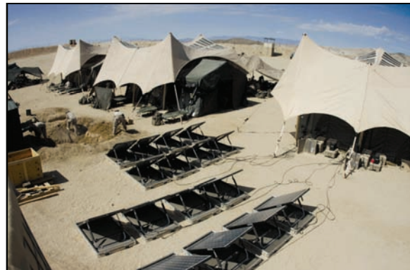
Solar array at a forward-operating base
